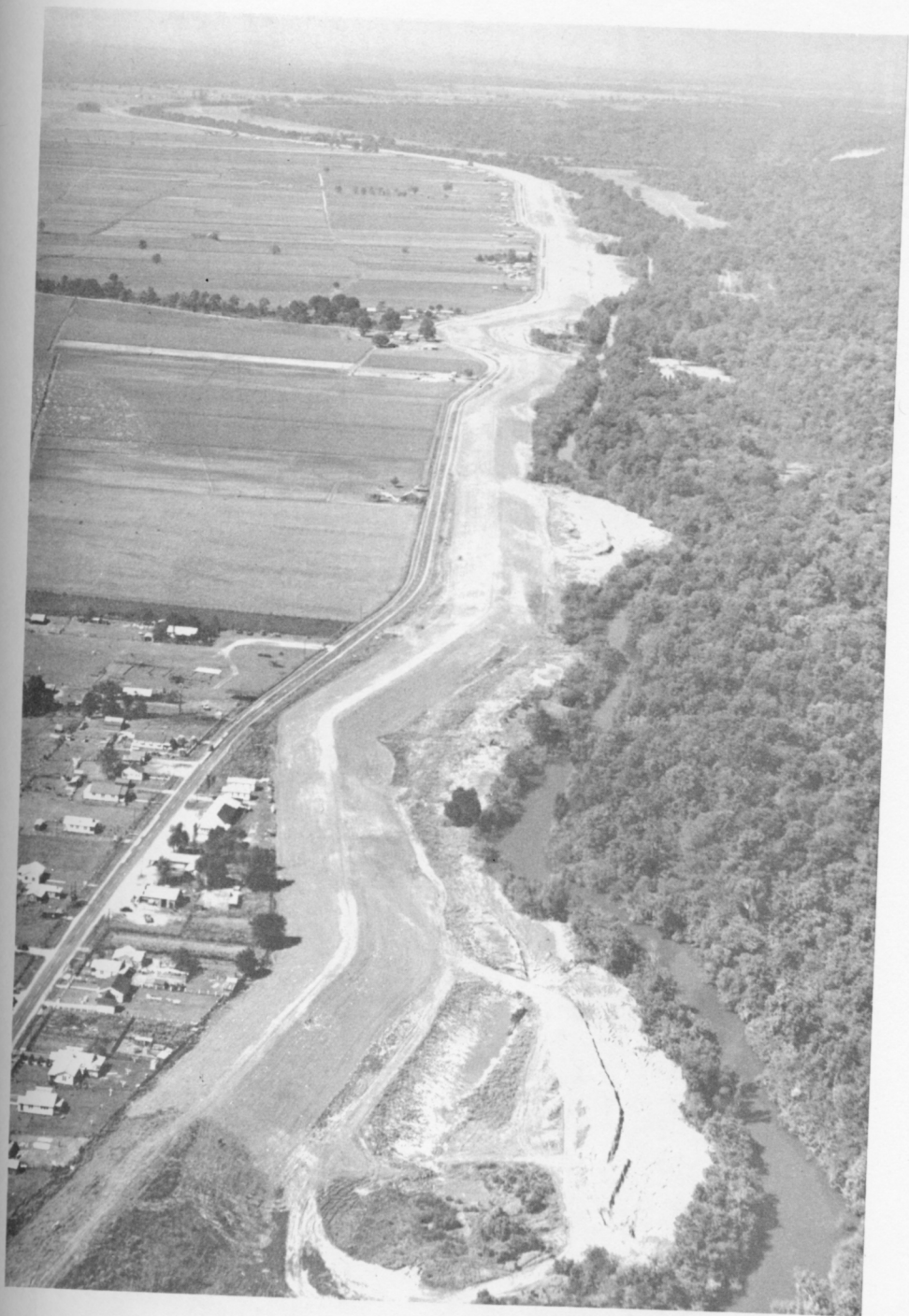
COURTESY OF US C OF E WEST ATCHAFALAYA FLOODWAY ILLUSTR. 1 Portion Of Fuse Plug Levee At Head Of Floodway Between Simmesport And Hamburg
