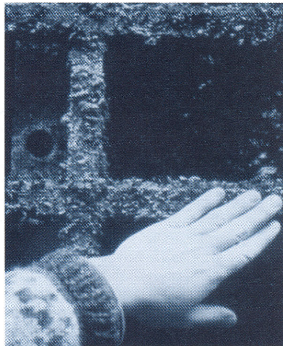
Zebra mussels have become a foulant for inland navigation by settling in towboat sea chests and keel coolers.
