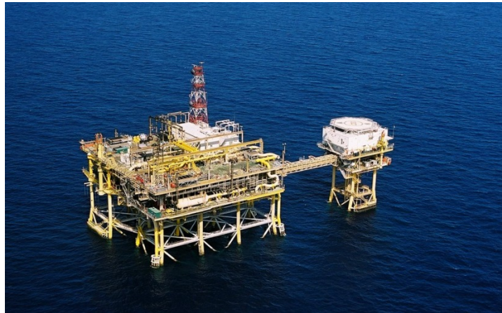
Figure 2.5: Louisiana Offshore Oil Port
