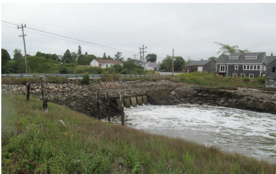
Water drains at low tide through a tidal restriction on the West Branch of the Pleasant River at Addison, Maine.
