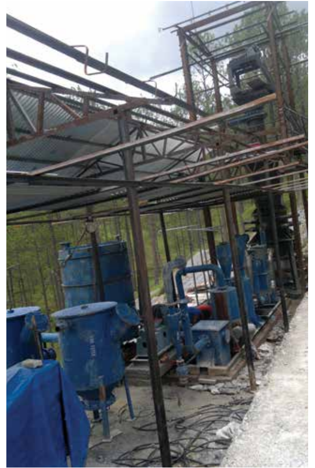
Pine needle gasifier under construction.
