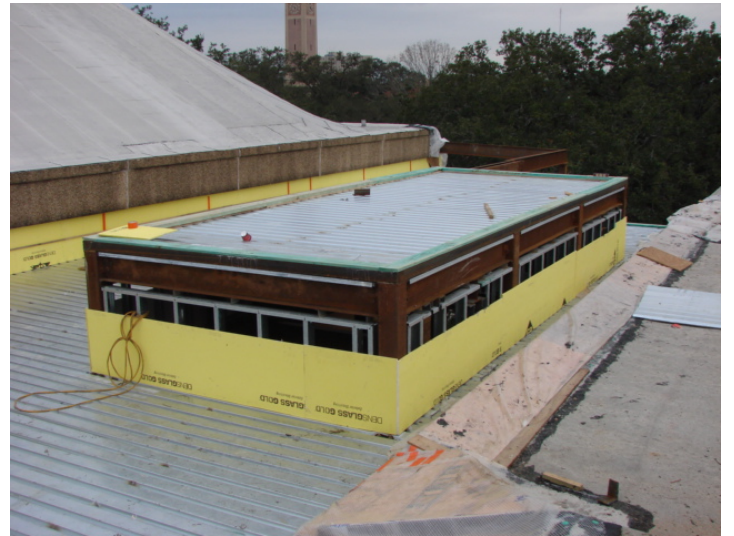
6. Shaft wall assembly for the two elevators in the connector.
