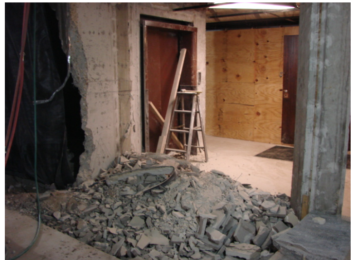
8. Demolition for the existing elevator continues on the 1 st floor.
