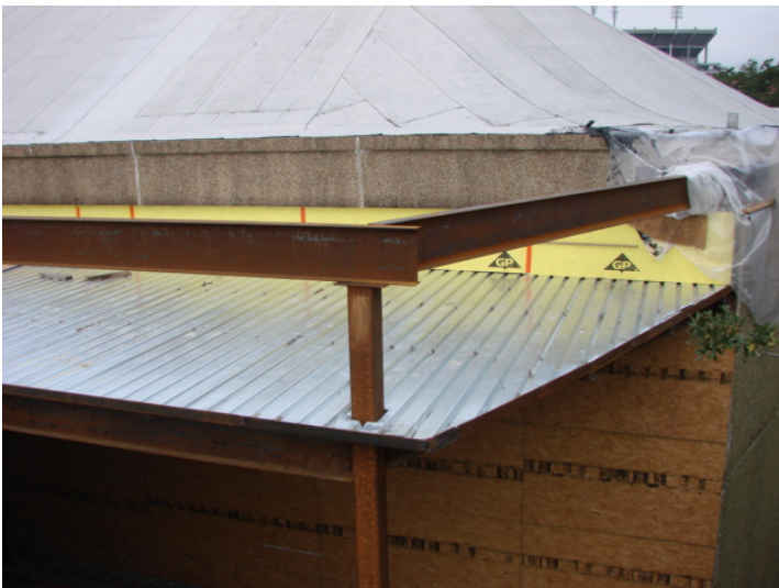
7. Roofing deck installed at the connector.
