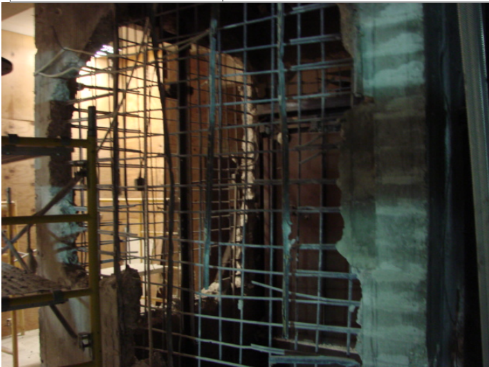
1. & 2. Existing concrete elevator shaft continues to be demolished on the third floor of the Union.
