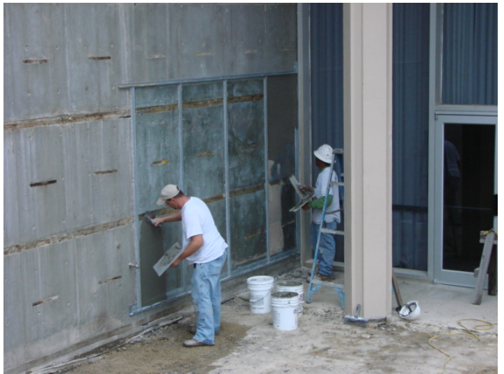
12. Work begins on the exterior aggregate plaster mock up.
