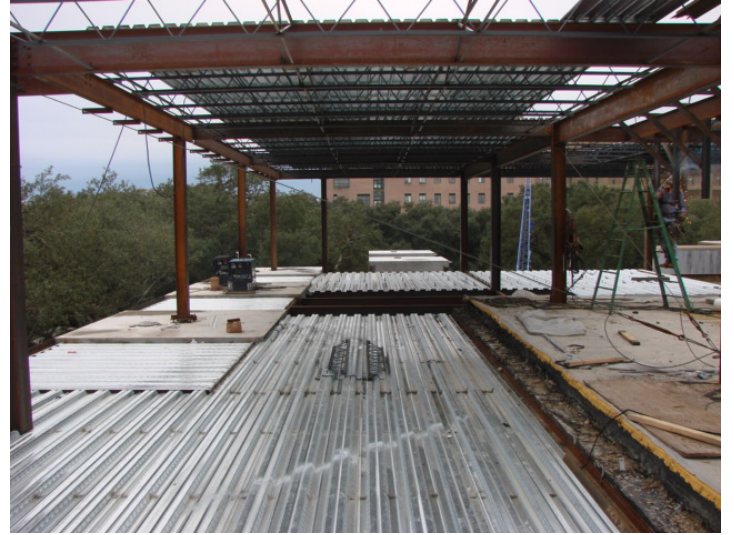
3. & 4. Metal decking and structural steel work continued on the third and fourth floors of the new S.E. addition.
