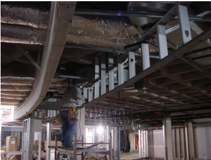
11. Metal stud ceiling work continues in the commons lounge.
