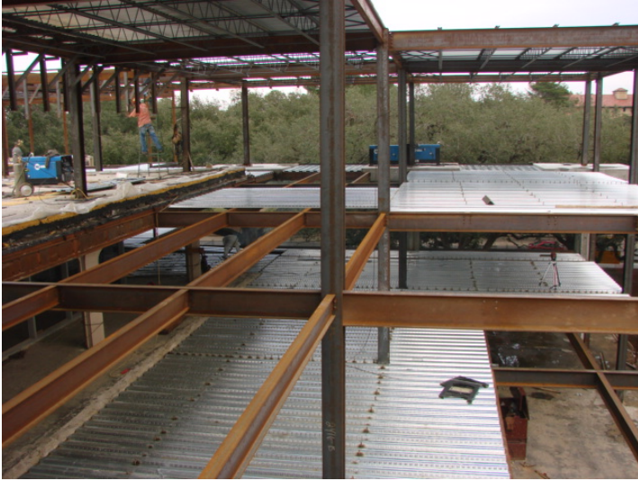
3. & 4. Metal decking and structural steel work continued on the third and fourth floors of the new S.E. addition.
