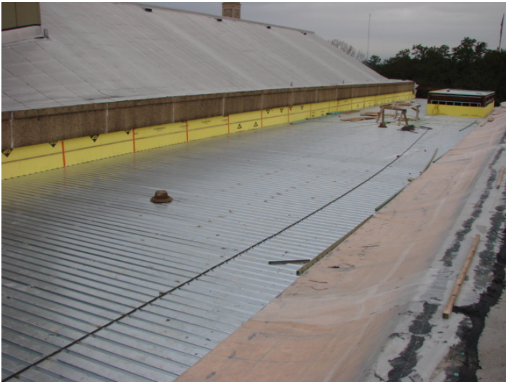
5. Roof decking continues to be applied to the connector.
