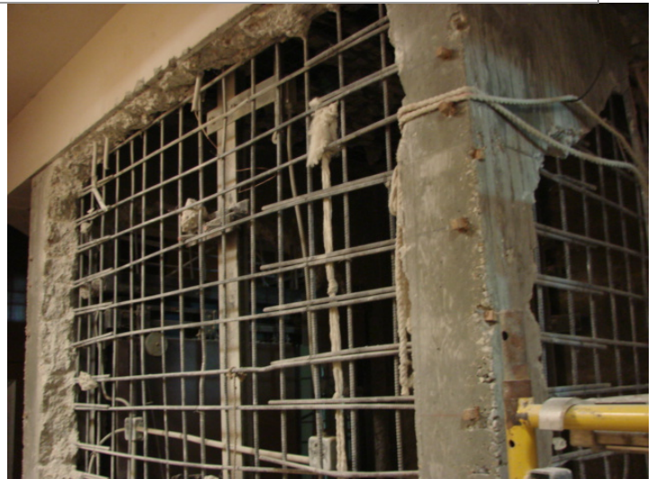
1. & 2. Existing concrete elevator shaft continues to be demolished on the third floor of the Union.
