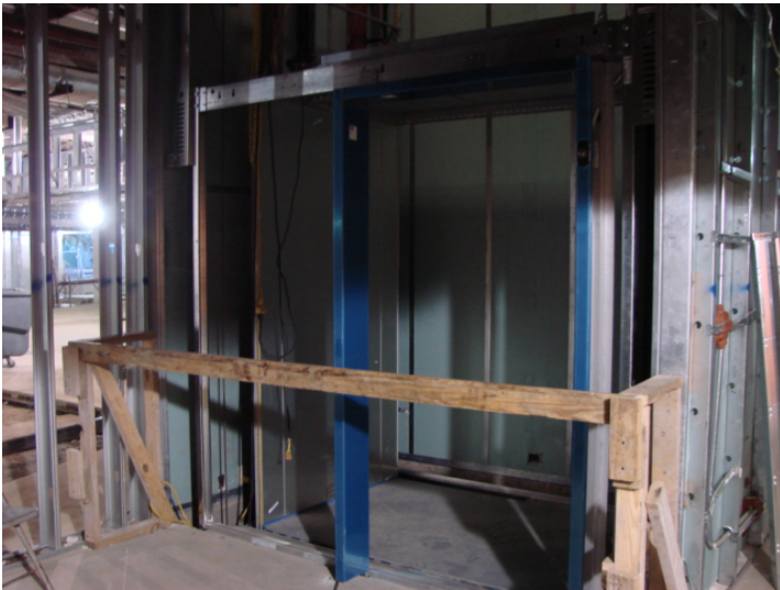
5. Work continues on elevator E103.
