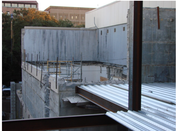
6. Concrete demolition continues at the existing cooling tower.
