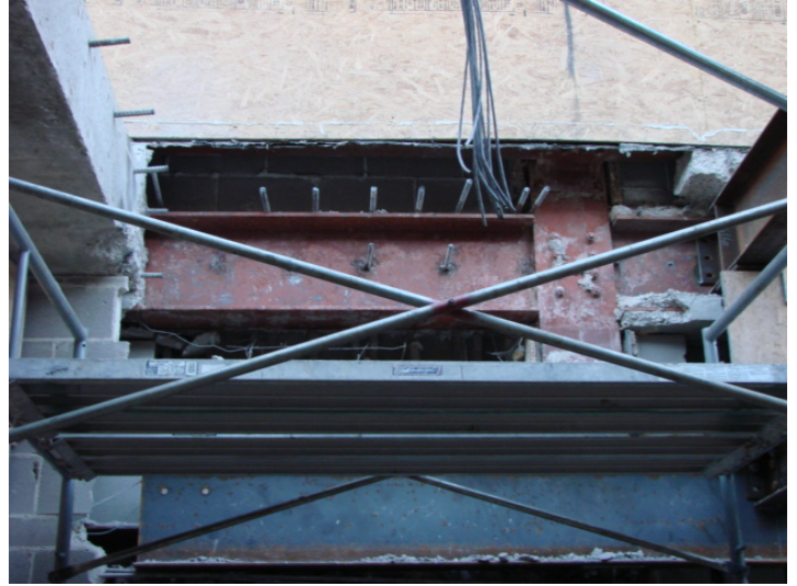
10. Demolition work at the existing wall of the theater.
