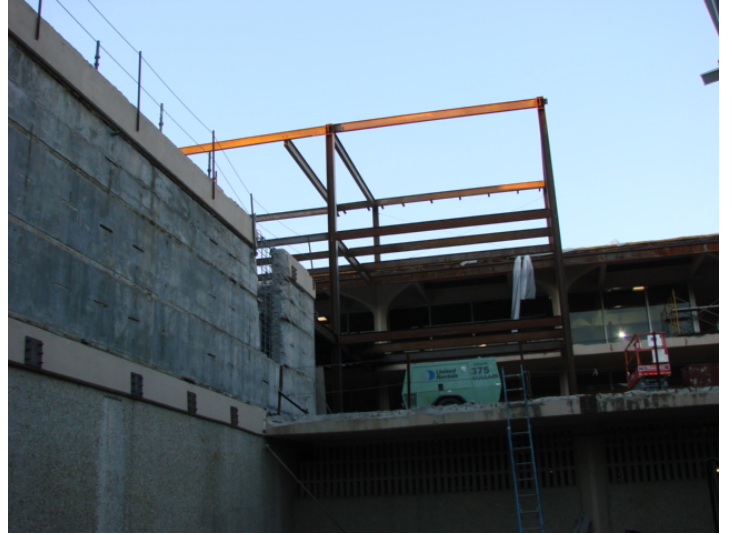
4. Structural steel erection continues at the S.E. addition.
