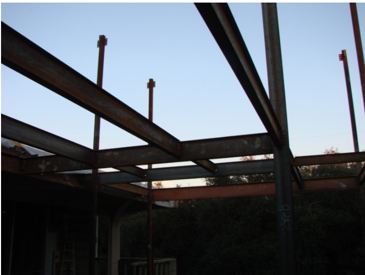
7. & 8. Structural steel erection continues at the southeast addition and around the tree columns.
