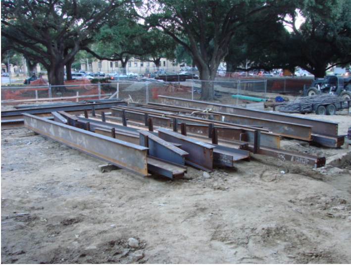
3. Structural steel waiting to be set in place at the southeast.
