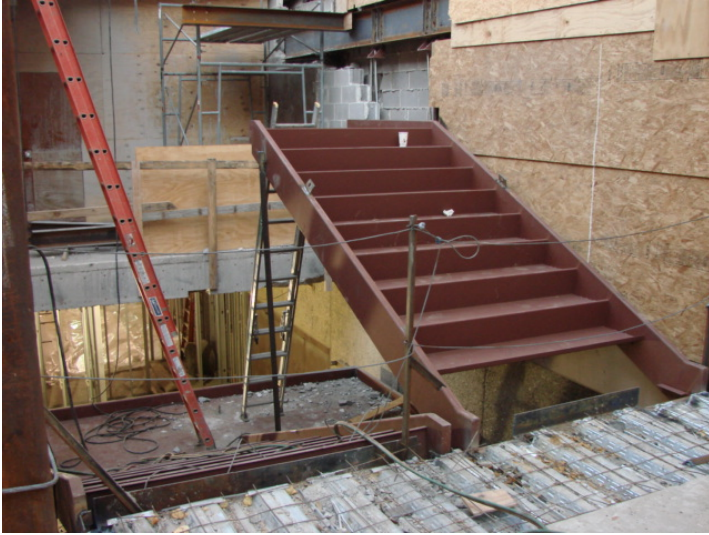
9. Metal stairs in place near the north end of the connector.
