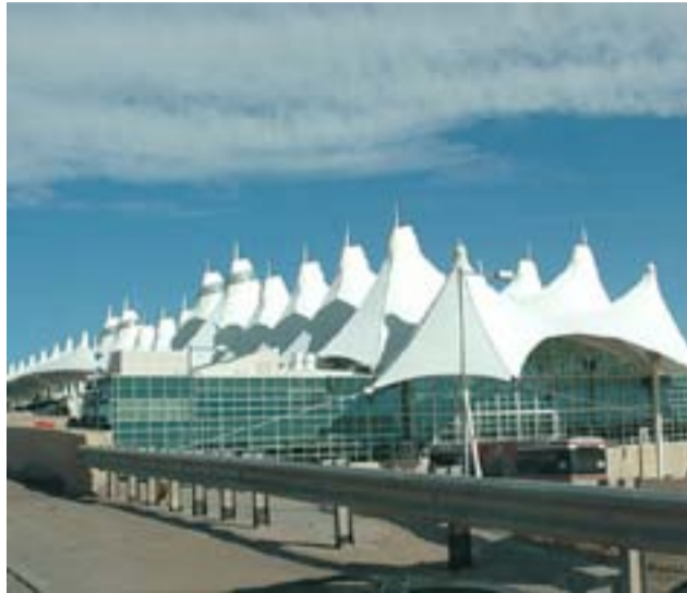
Denver International Airport
