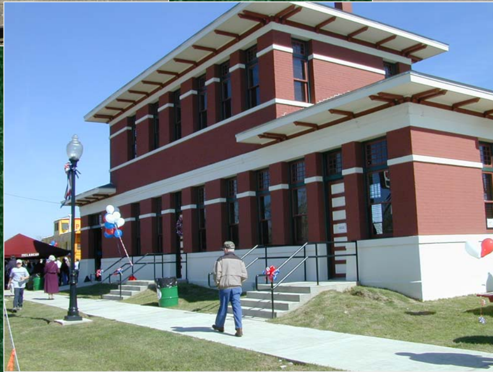
Bunkie Train Depot
