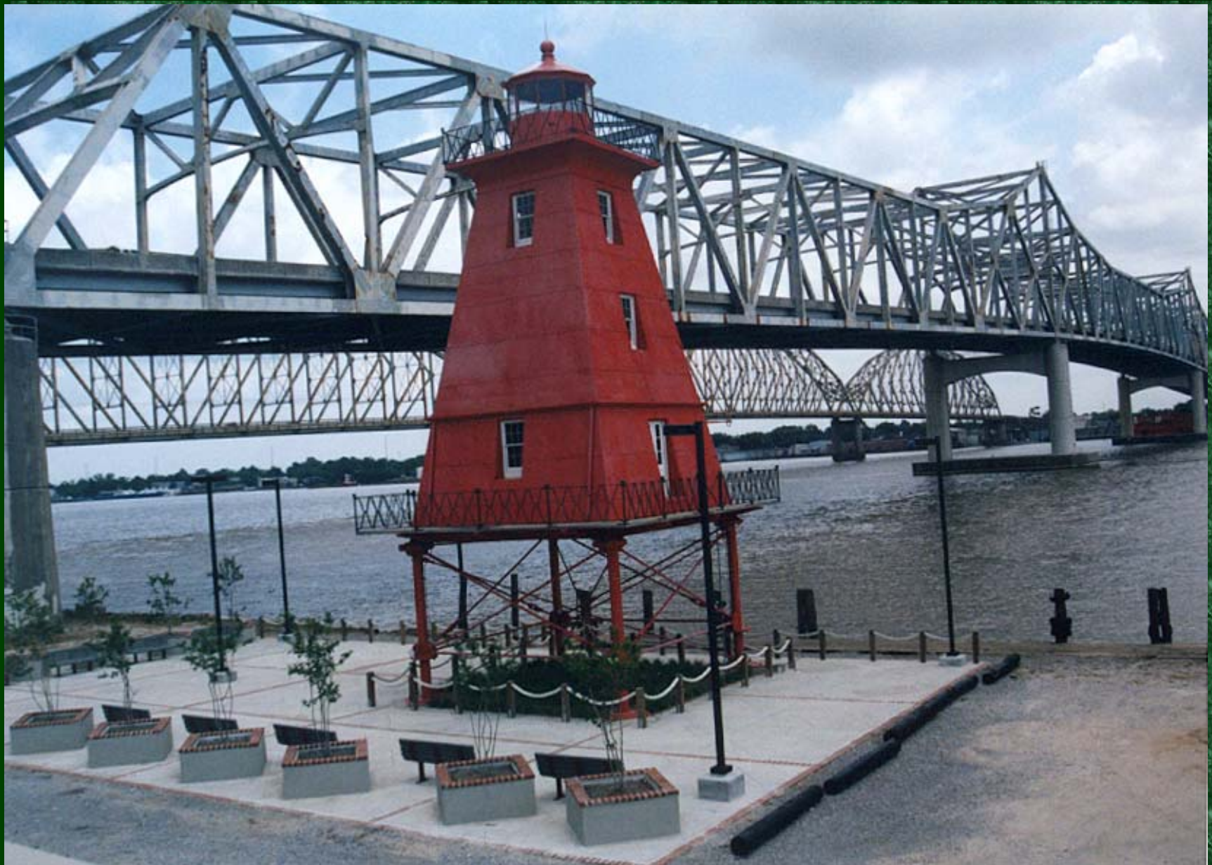
Berwick Lighthouse Restoration
