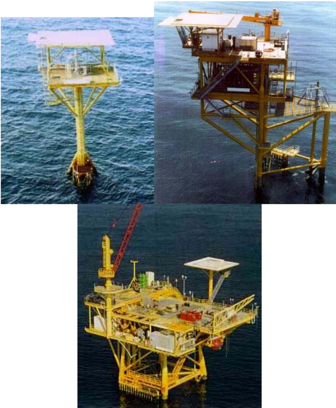
**Figure A.2. Caisson, Well Protector, and Fixed Platform Structures
